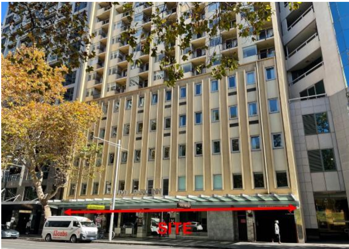
Figure 5: Site's frontage to Elizabeth Street
